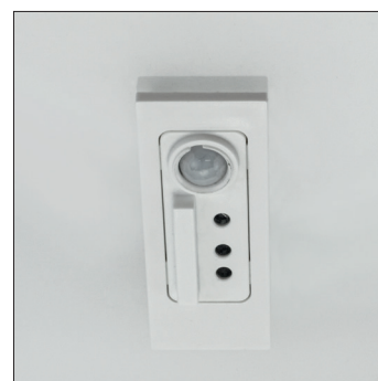
XC daylight&occ sensor
